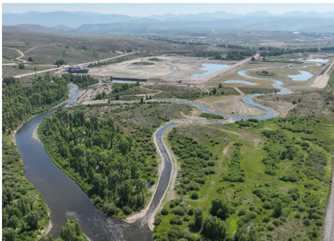
The Colorado River Connectivity Channel was completed in 2024.
