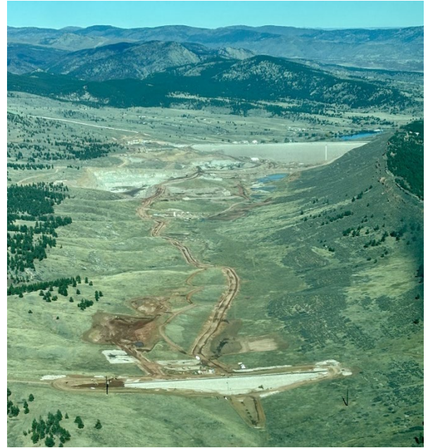
Aerial view from the south end of the Chimney Hollow Reservoir project showing the saddle dam in the foreground and the main dam in the background.
